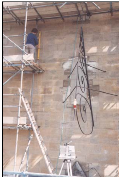
Fig. 7. John Davis' invention for aligning the gnomon
