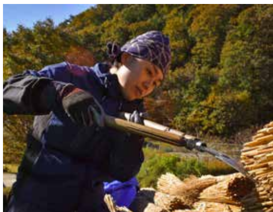
Saori shearing eaves
