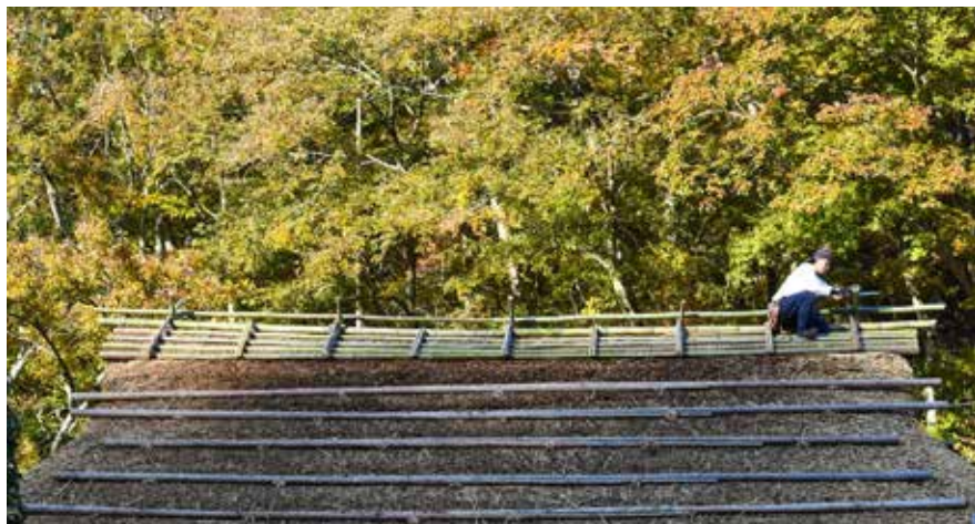
Saori Ohno finishing thatching of ridge, Japan
