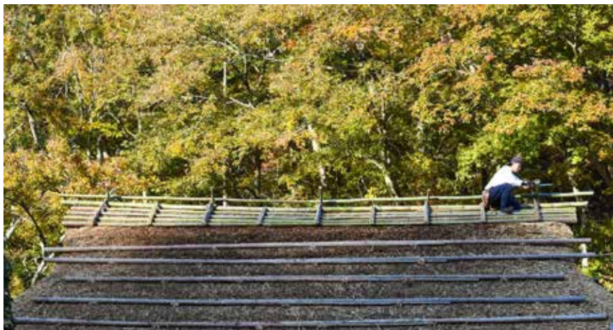
Saori Ohno finishing thatching of ridge, Japan
